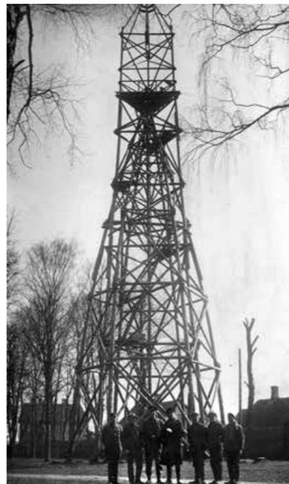
In 1931 for observation purposes a 42 m high triangulation wooden tower was built above the Struve point. For several summers, the teaching staff and students of the University of Latvia conducted astronomical and geodetic research and measurements
